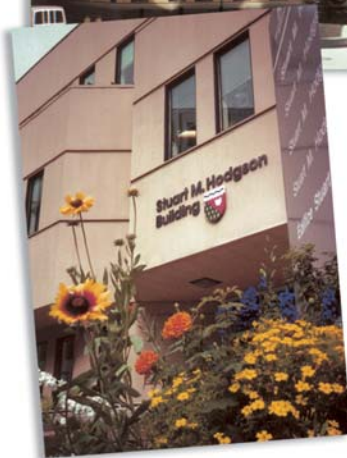
The 2nd floor of the Stuart M. Hodgson Building in Yellowknife houses the GNWT's headquarters data centre and communications network, and Systems and Communications Division staff.
